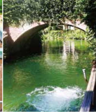
▶ Water circulation and oxygen supply : installed at one meter depth
